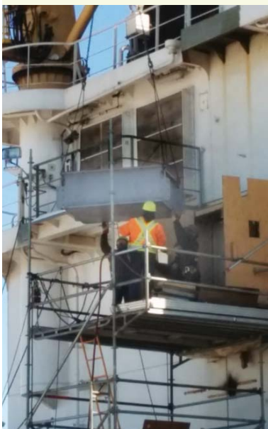
A Membrane Scrubber module is ready to be put inside the Baie St. Paul’s funnel.
